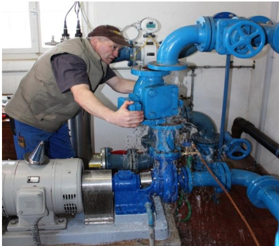
Fountainmaster Gysin removes the old check flap
