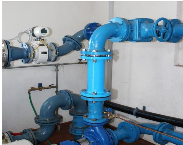
Mounting the Stop Silent valve in between the flanges
