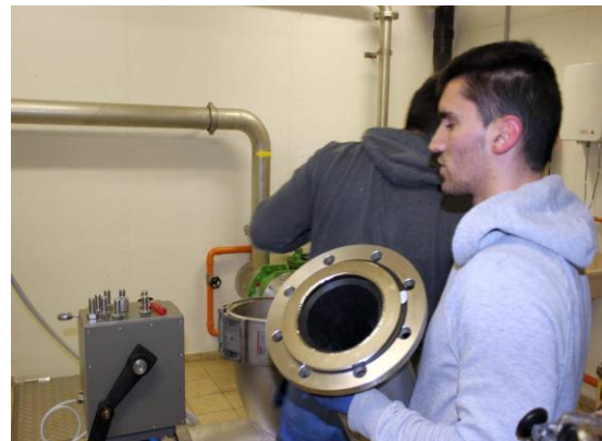
AS54 check valve inserted in pipe
