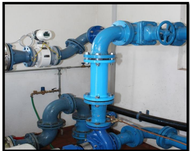
Mounting the Stop Silent valve in between the flanges
